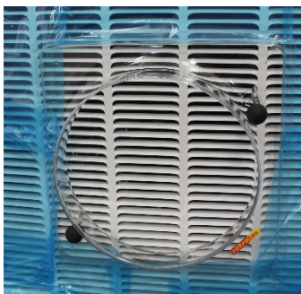
Figure 19: Flange taped onto a return register before attaching the Flex Duct
