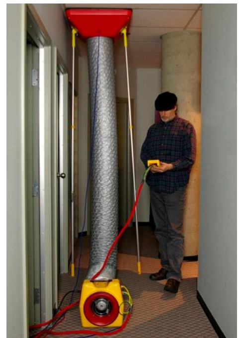
Figure 40: Measuring air flow with a Powered Flow Hood
