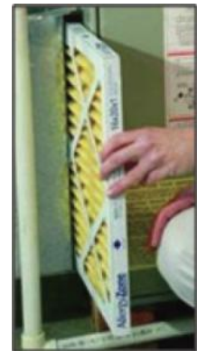
Figure 11: Remove all air filters
