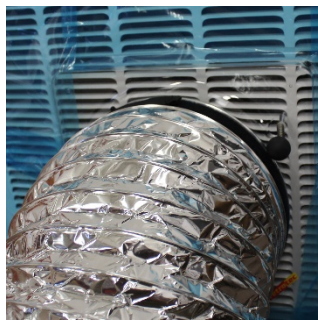
Figure 18: Flex Duct connected to the Flange.
