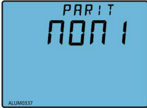
Fig.3-39 communication check setting
