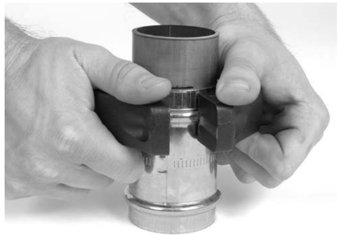
Figure 8 – Installing Press Ring Onto Fitting
