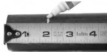
Figure 6A – Marking the Pipe Before Inserting Into Fitting Using Tape Measure
