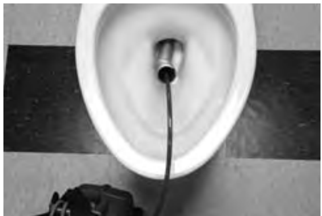
Figure 25 – Using The Flexible Guide Tube
