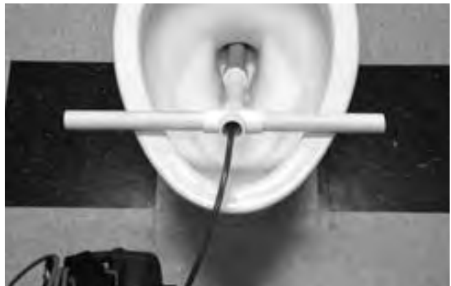
Figure 24 – Using A PVC Guide Tube
