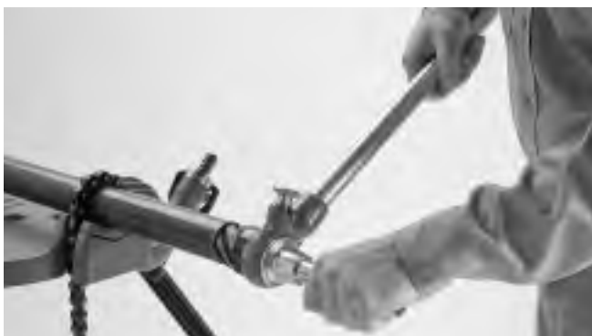
Figure 2 – Reaming End of Pipe
