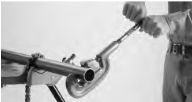
Figure 1 – Cutting End of Pipe
