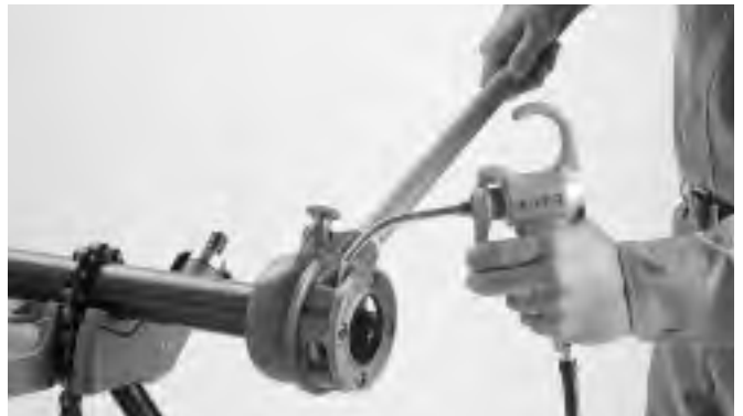
Figure 4 – Applying Thread Cutter Oil
