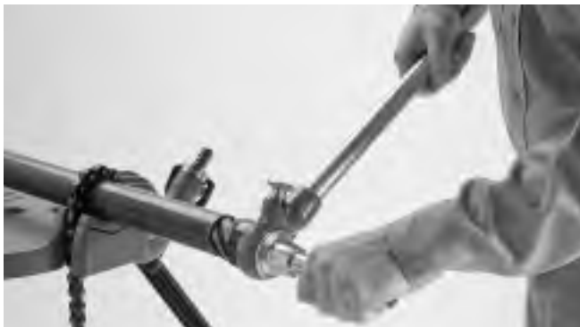
Figure 2 – Reaming End of Pipe
