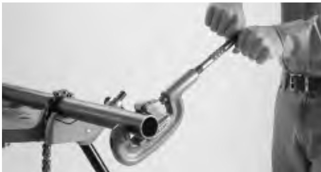
Figure 1 – Cutting End of Pipe
