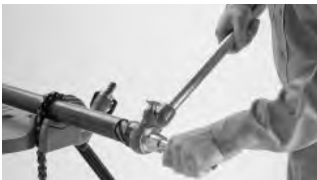
Figure 2 – Reaming End of Pipe
