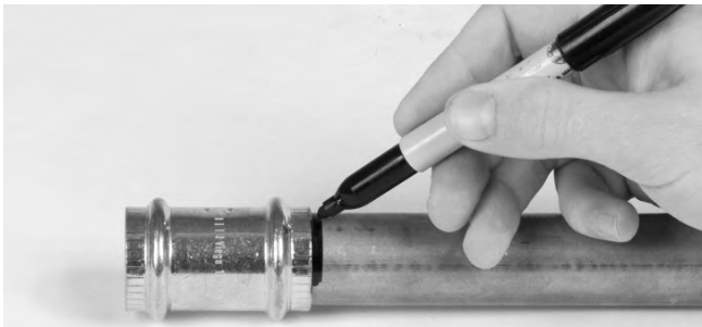
Figure 8 – Marking the Tubing After Fully Inserting Tube
